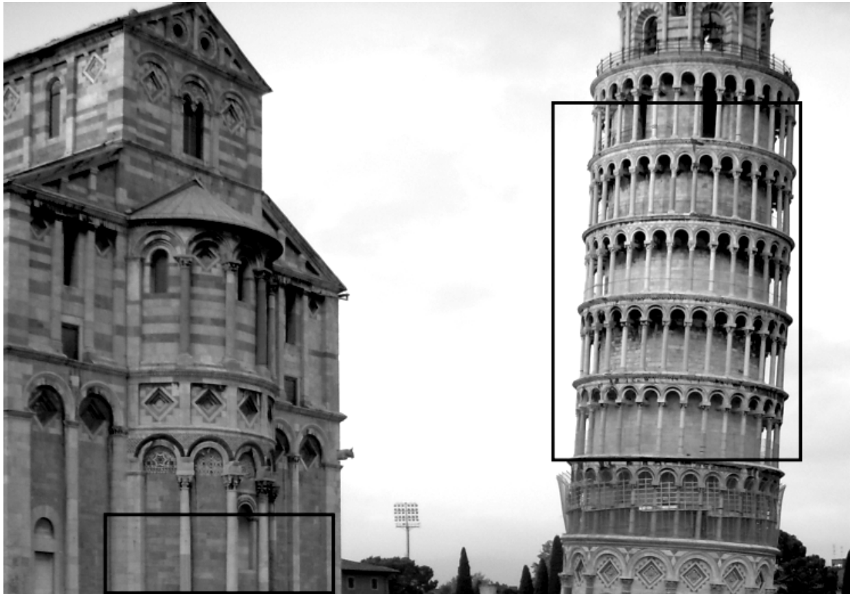
Figure 3. Pisa Tower. The chosen parts of the image are separated by rectangles.
